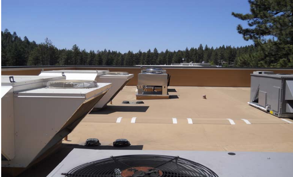
Roof and HVAC
